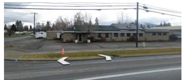
Building demolished as part of Marketplace at Miles OPA
