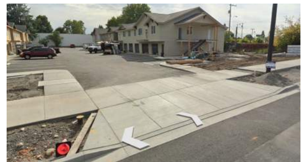
Frontage improvements constructed as a part of the Chubbs OPA
